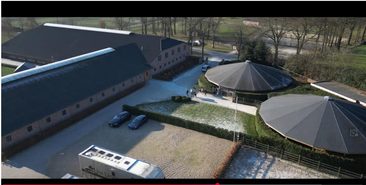
Covered walker and covered longeing ring
